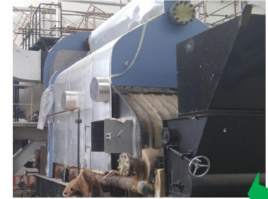
Biomass boiler: Produce high pressure, high temperature steam for hydrothermal reactor
